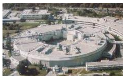
Elettra, Italy (2009) 2 GeV
